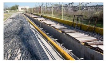
Fig. 1. Copper cable replacement
